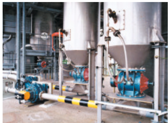
Product feed from silo via rotary valve.
